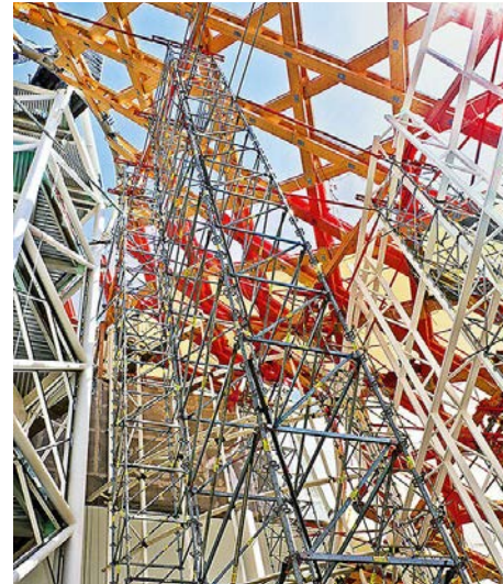
Fig. 14: Photo of the supporting tower
