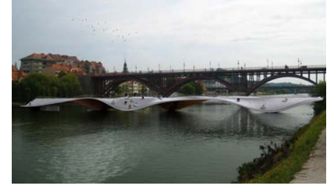
Fig. 8: Photo of bridge
