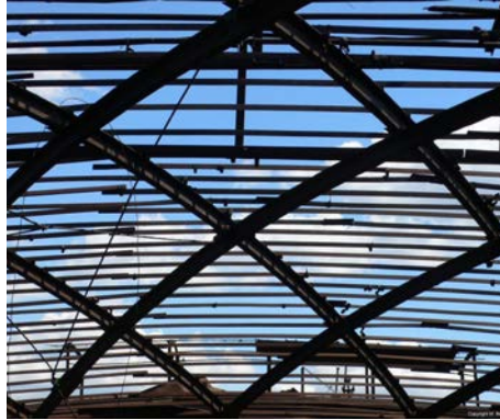
Fig. 7: Detail of Z-shaped steel structure
