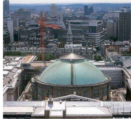
Fig. 14: Photo (before the construction)
