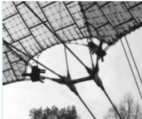
Swaged clamp connection
