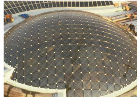
Fig. 14: The top view of the dome
