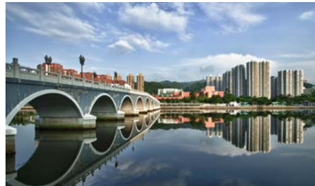
b. Shatin Central Park Bridge
