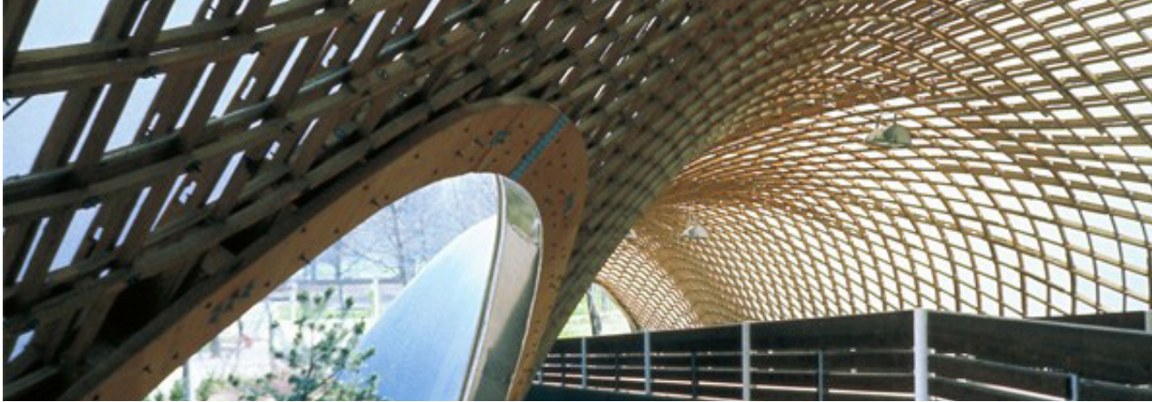
Fig. 2: Multihalle, Mannheim, Germany
