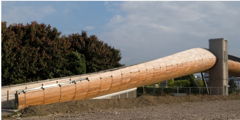
Fig. 13: Photo of footbridge
