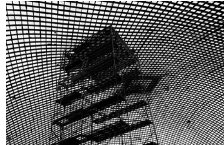
Fig. 13: Photo of Multihalle interior
