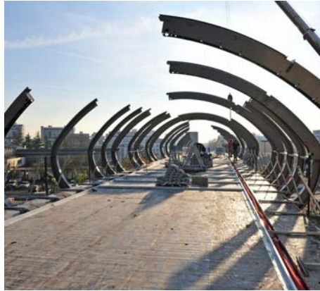
Fig. 11 & 12: Photos of footbridge
