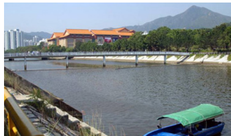
c. Shing Mun River Bridge
