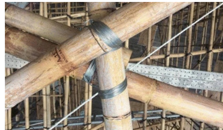
Fig. 4d Photo of the joints
