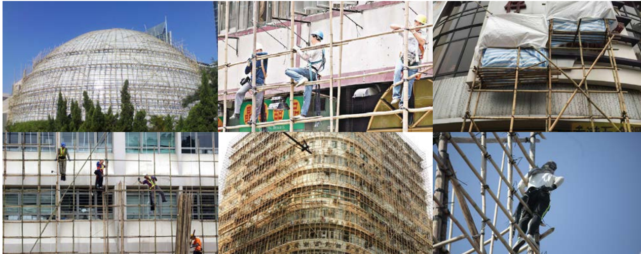
Fig. 1: Bamboo scaffolding in Hong Kong
