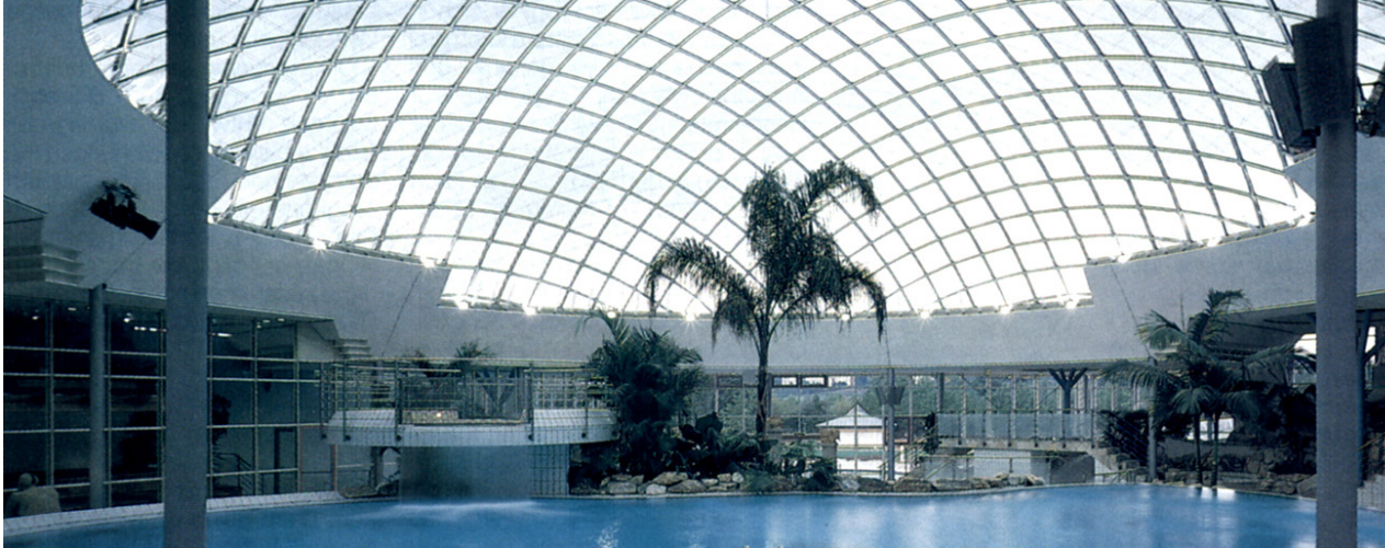
Fig. 1: The interior of Aquatoll Neckarsulm
