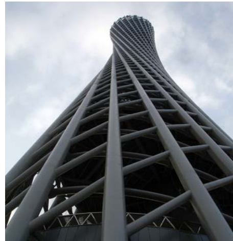
Fig. 7: Facade of the building
