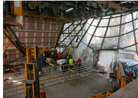
Fig. 13: Photo of construction
