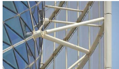
Fig. 7: Typical joints and supports
