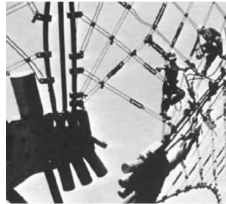
Fig 14: Erection of cable networks
