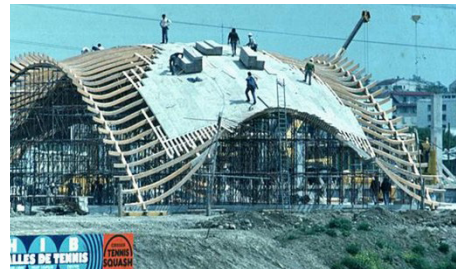
Fig. 10: Timber formwork
