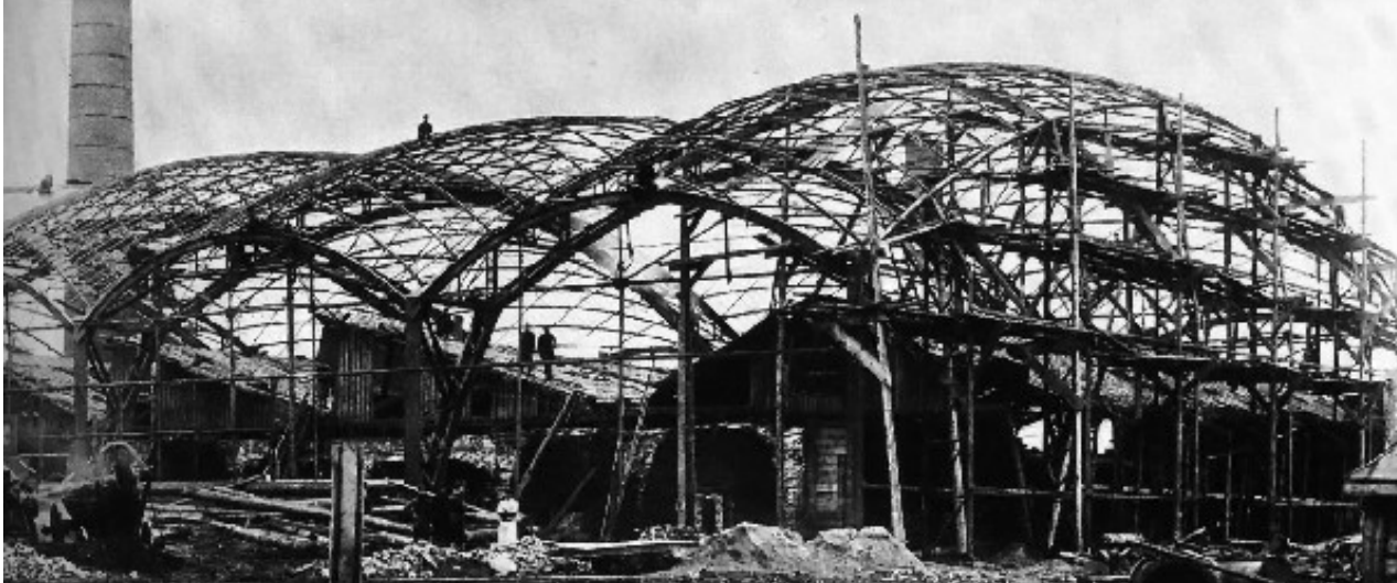
Fig. 1: Production Hall by Vladimir Shukhov in Vyksa
