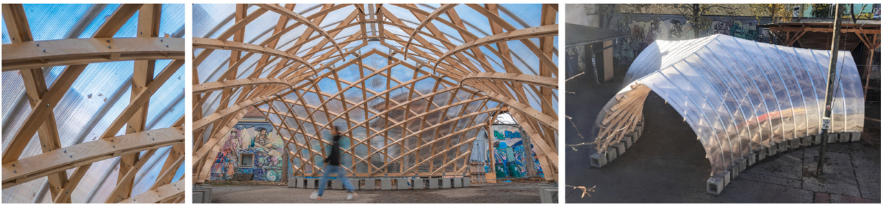
Fig. 3. The Asymptotic Geodesic Hybrid Gridshell. Three timber shells are joined to create a negatively curved gridshell. The structure is covered with polycarbonate panels along the geodesic directions. (Photos: Yilinke Tan).
